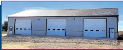
Ag Building 60' x 100' Equipment Storage
