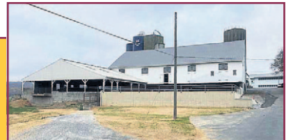
NRCS project in Penryn, PA (After)
