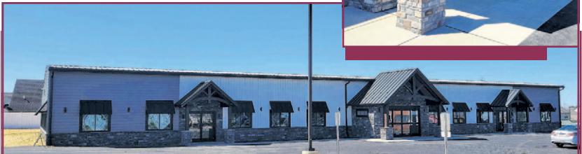
Commercial Building Remodel - (After)
