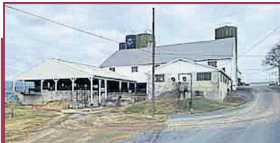
NRCS project in Penryn, PA (Before)
